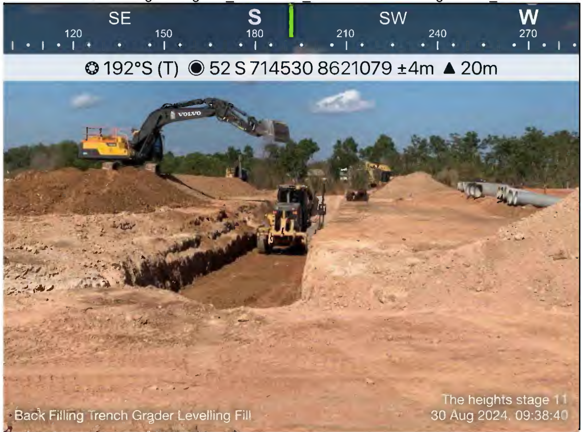
e heights stage 11_2024-08-30_Back Filling Trench Grader Levelling
