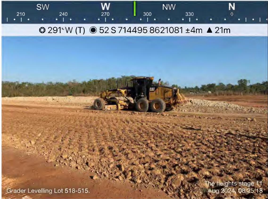
- The heights stage 11_2024-08-30_Grader Levelling Lot 518-515_
