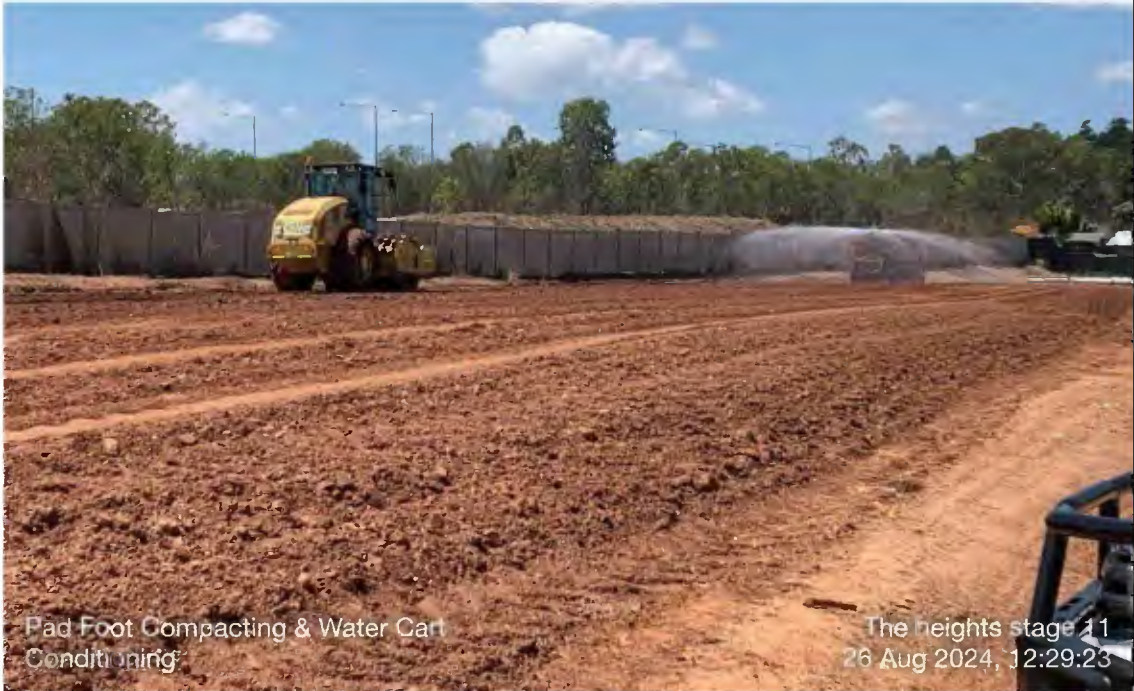
hts stage 11_2024-08-26_Pad Foot Compacting & Water Cart Conc
