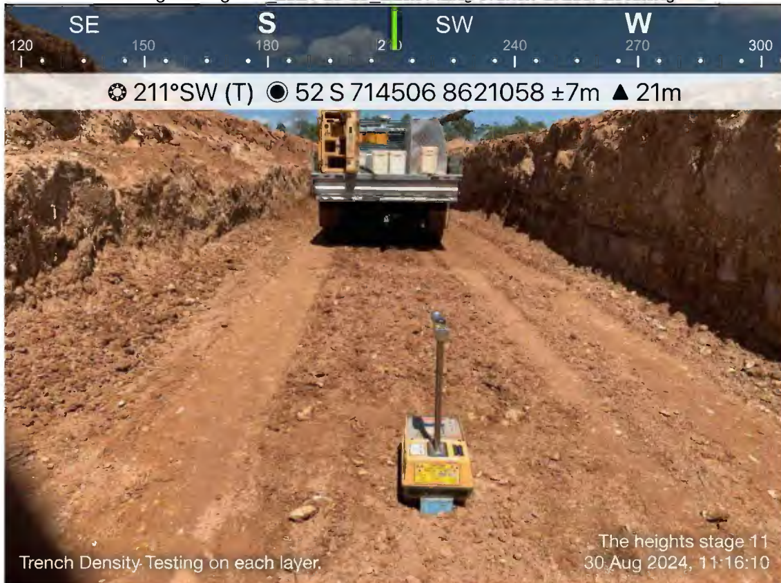
the heights stage 11_2024-08-30_Trench Density Testing on each lay
