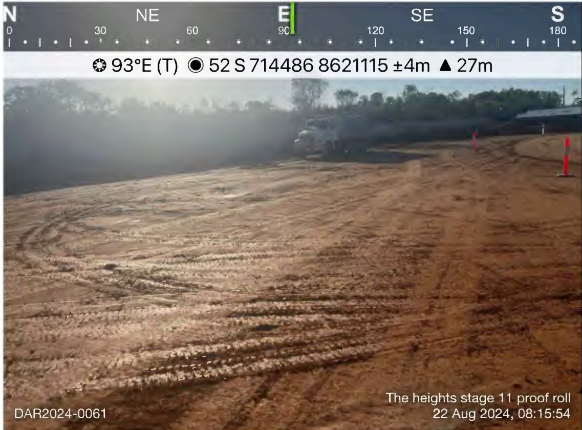
Photo 13 - The heights stage 11 proof roll_DAR2024-0061 3
