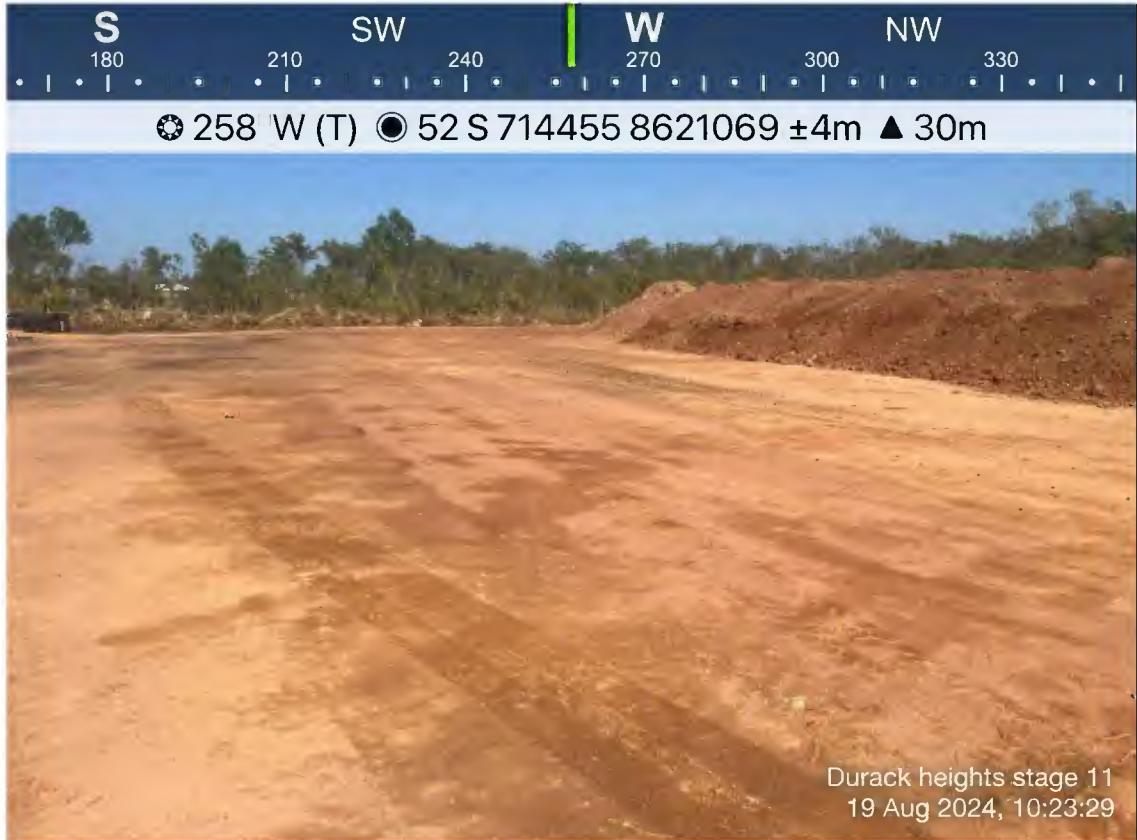
Photo 1 - Durack heights stage 11
