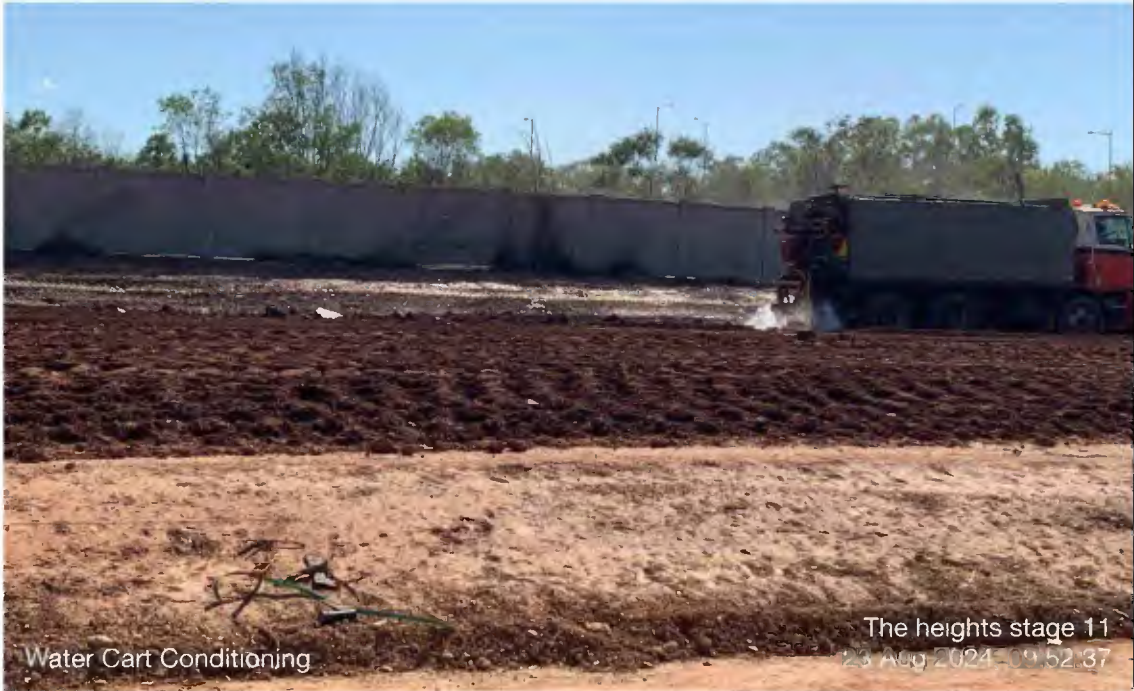
2 - The heights stage 11_2024-08-23_Water Cart Conditioning_09-
