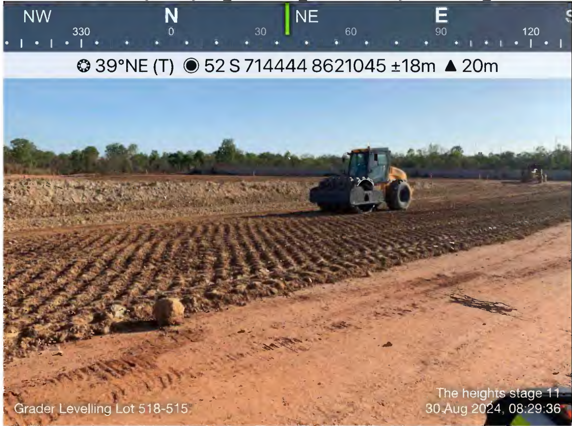
- The heights stage 11_2024-08-30_Grader Levelling Lot 518-515._
