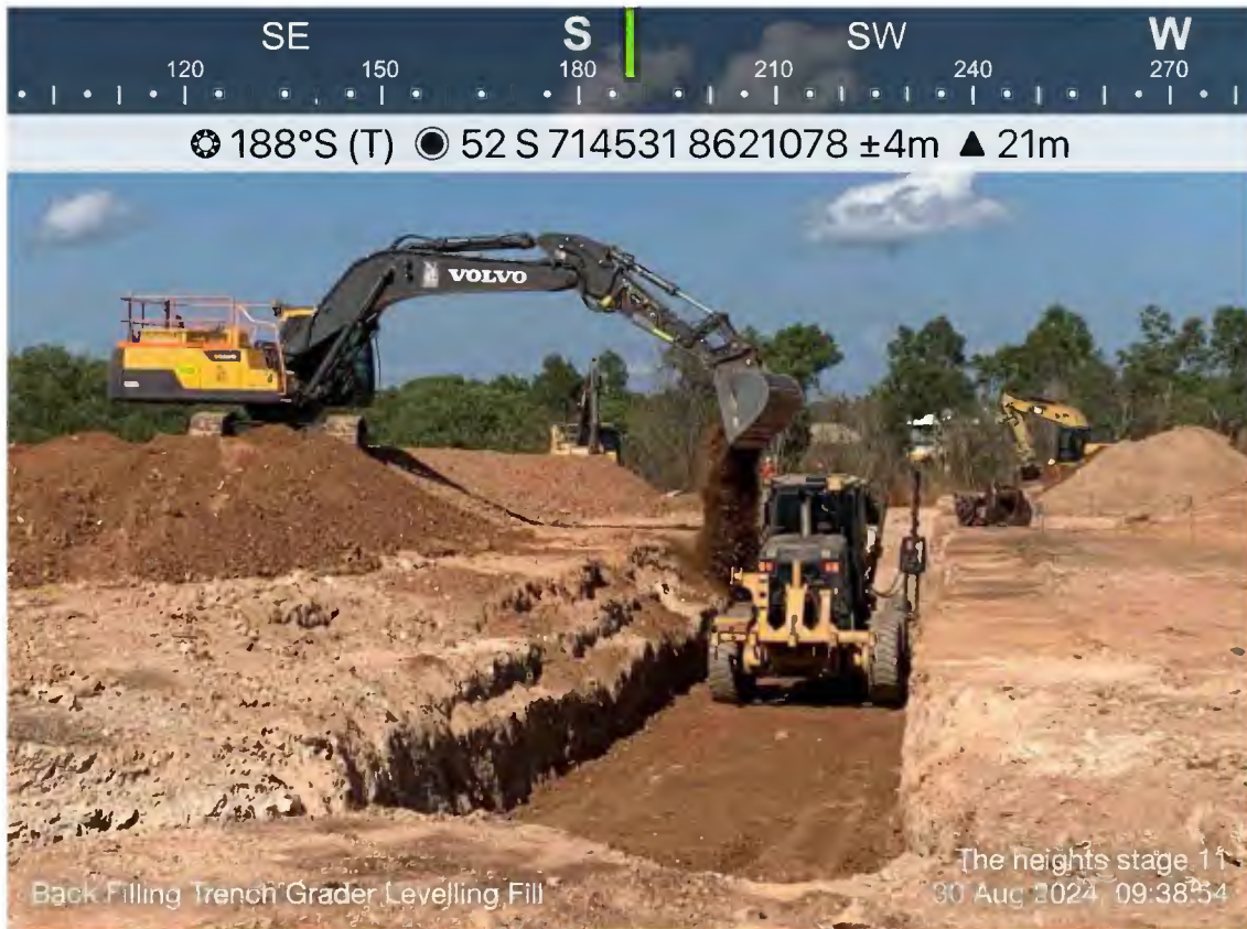
the heights stage 11_2024-08-30_Back Filling Trench Grader Levelling
