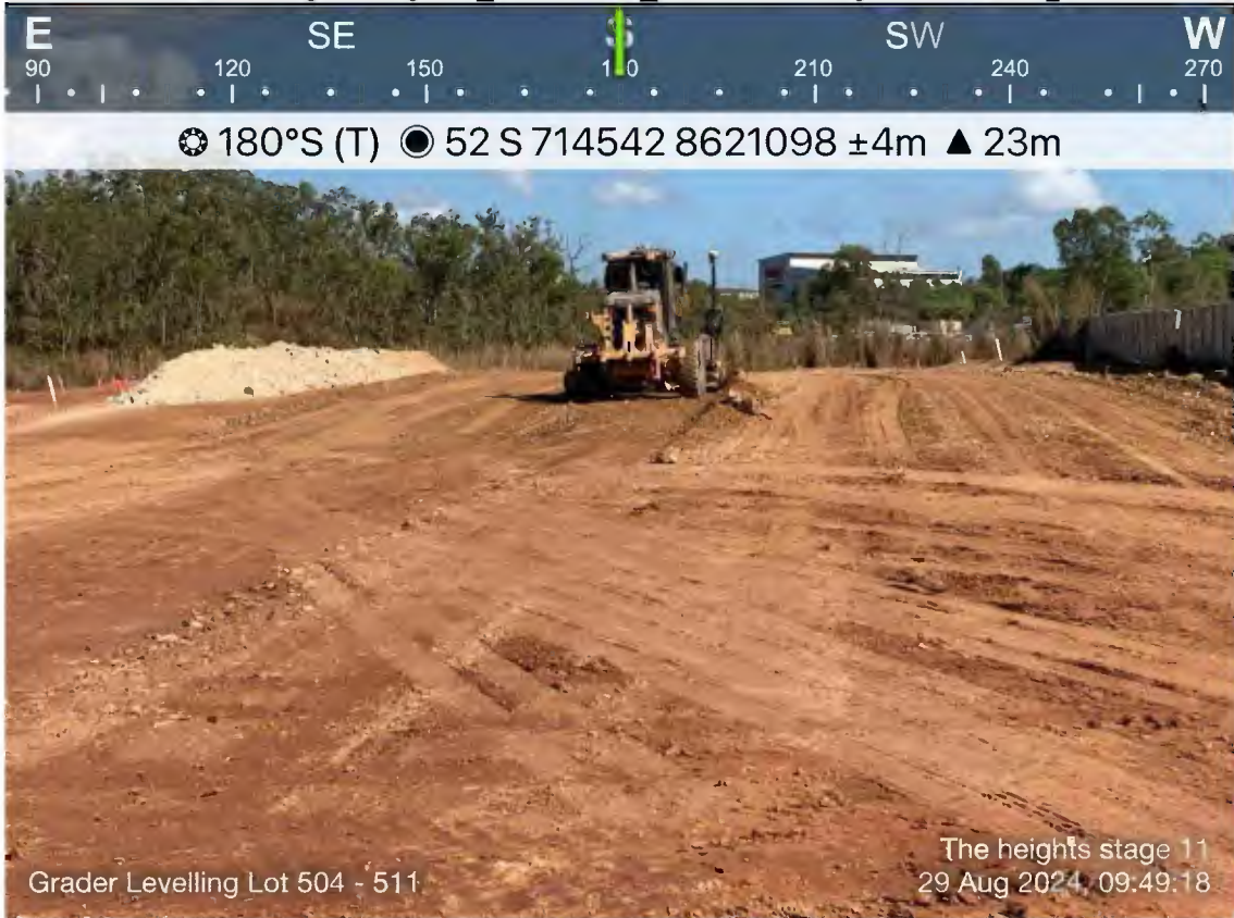
- The heights stage 11_2024-08-29_Grader Levelling Lot 504 - 511_
