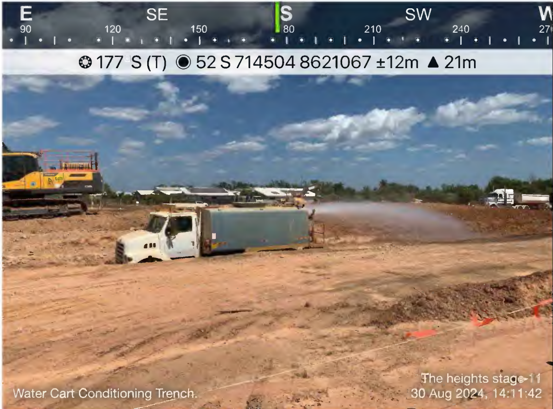
The heights stage 11_2024-08-30_Water Cart Conditioning Trench.
