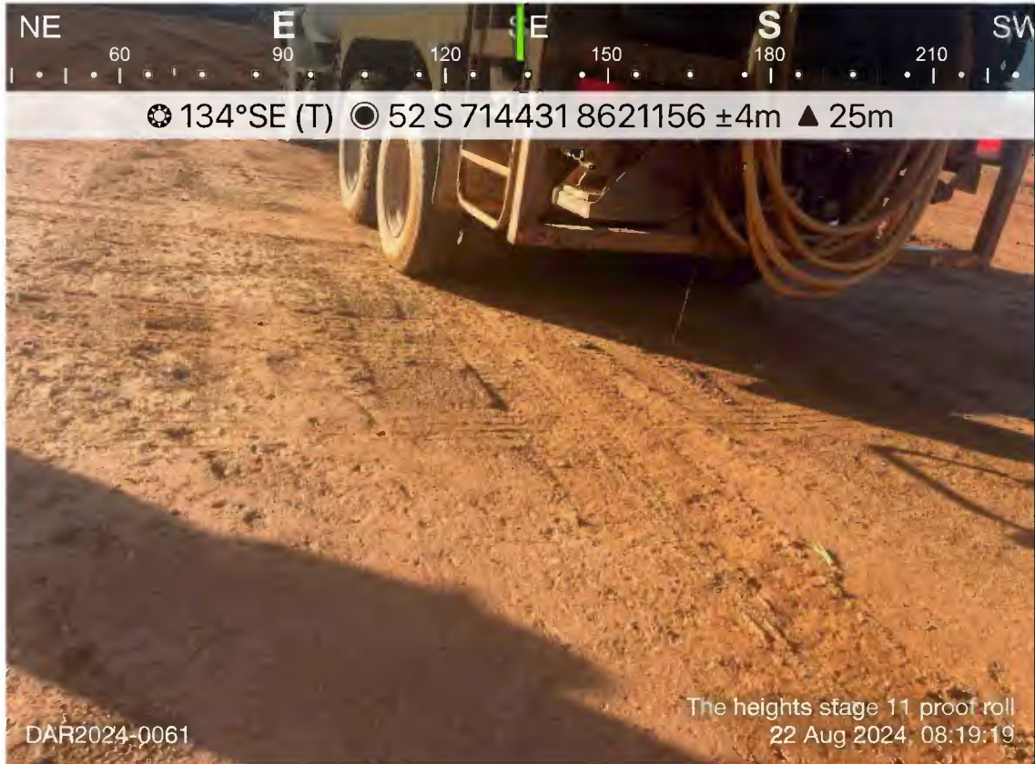
Photo 15 - The heights stage 11 proof roll_DAR2024-0061 5
