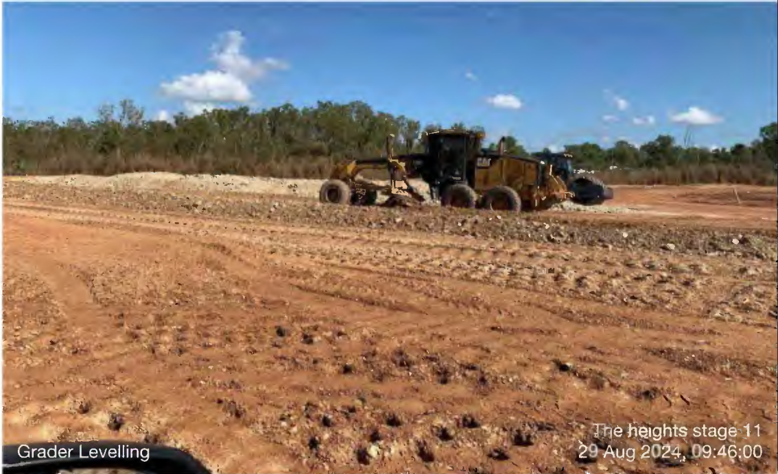
Photo 16 - The heights stage 11_2024-08-29_Grader Levelling_09-46-
