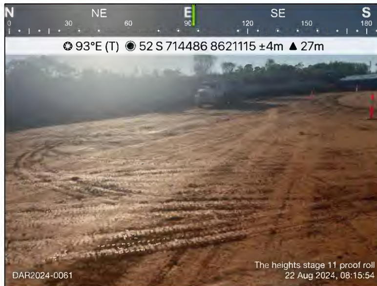
Figure 5: Post Strip area for proof roll
