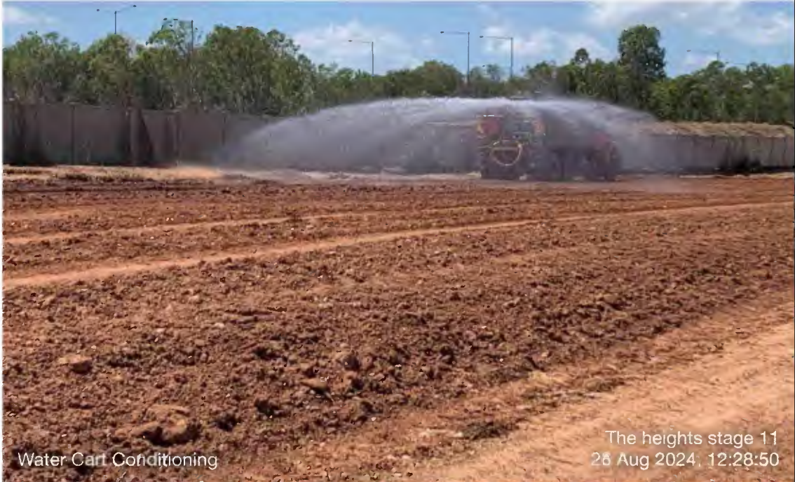
7 - The heights stage 11_2024-08-26_Water Cart Conditioning_12-
