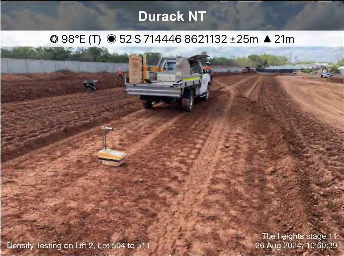
The heights stage 11_2024-08-26_Density Testing on Lift 2, Lot 504 to 511
