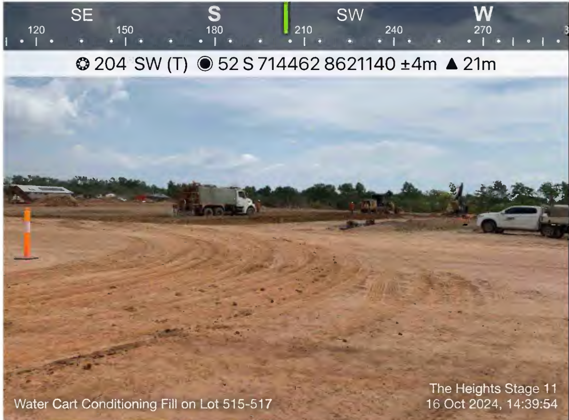
leights Stage 11_2024-10-16_Water Cart Conditioning Fill on Lot 515-517
