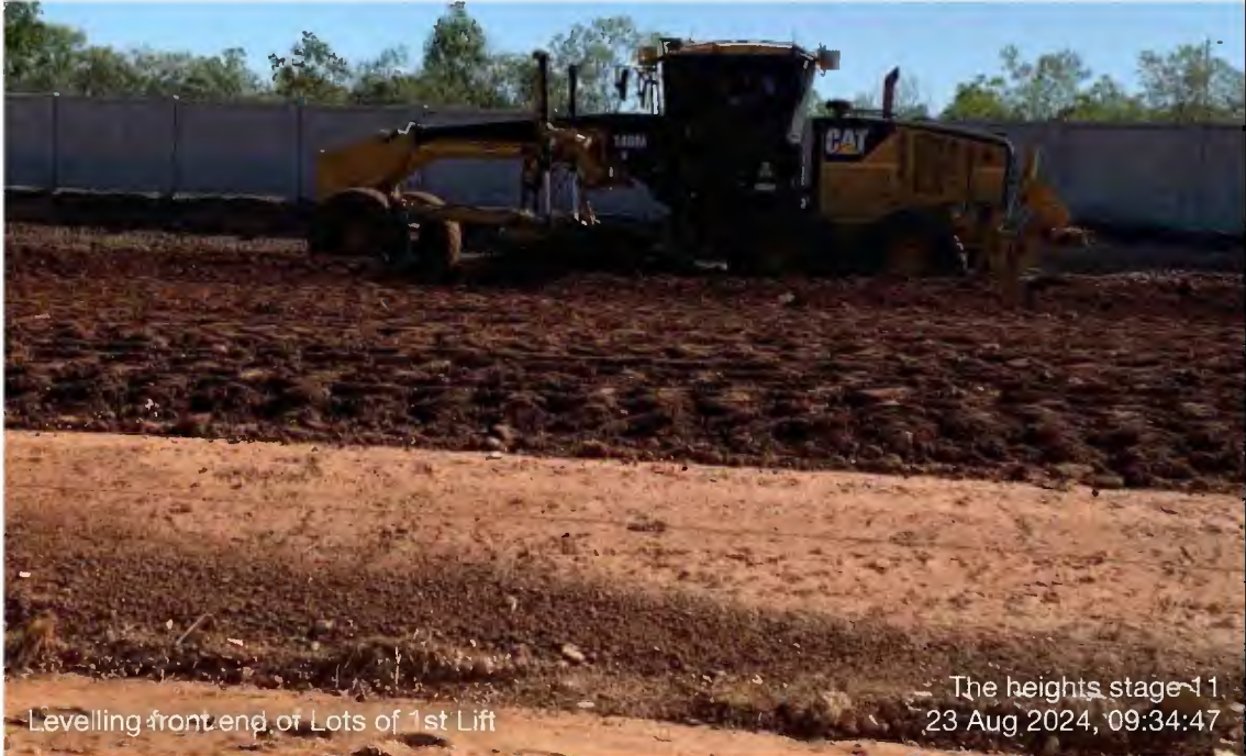
he heights stage 11_2024-08-23_Levelling front end of Lots of 1st Lift
