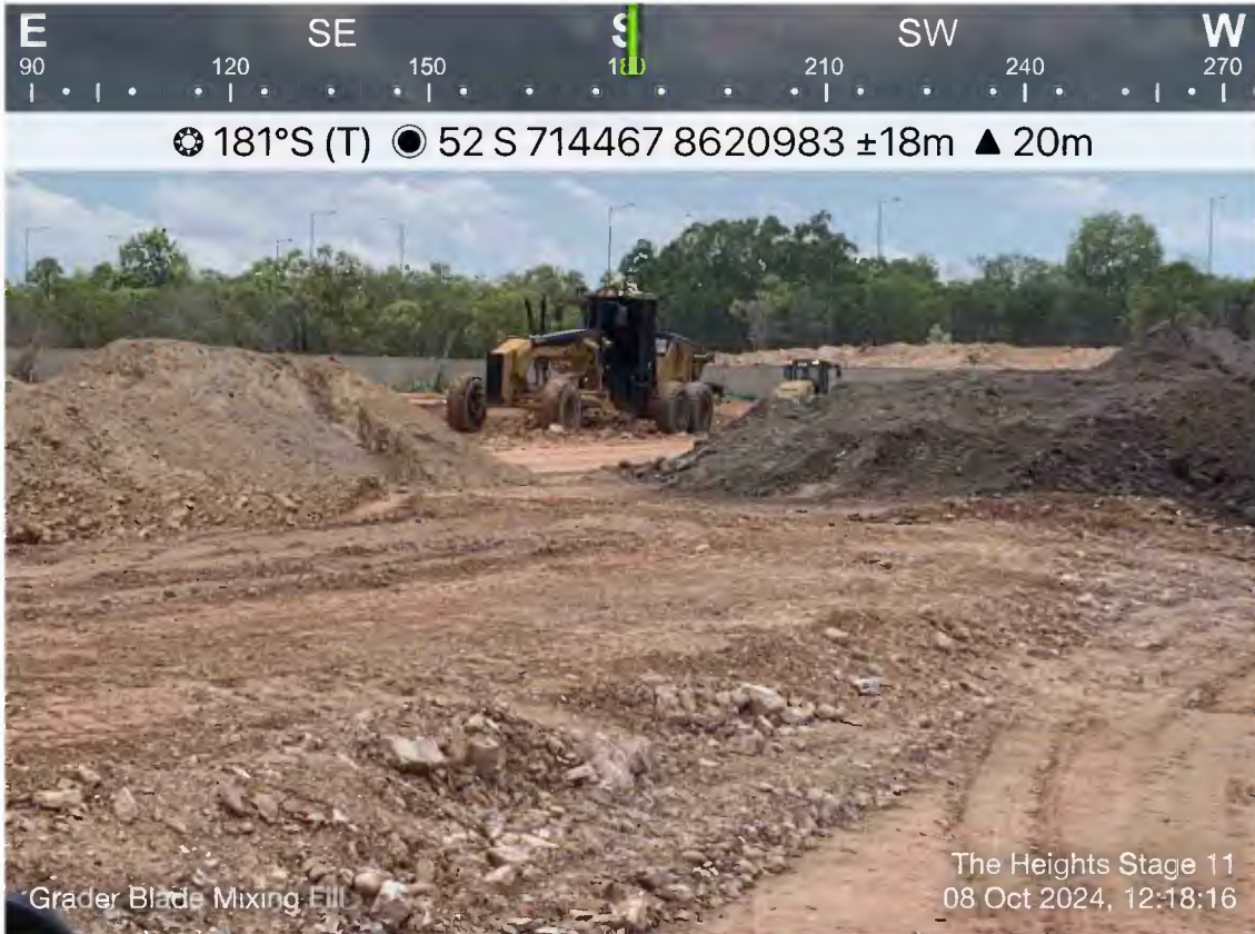
1 - The Heights Stage 11_2024-10-08_Grader Blade Mixing Fill_12-
