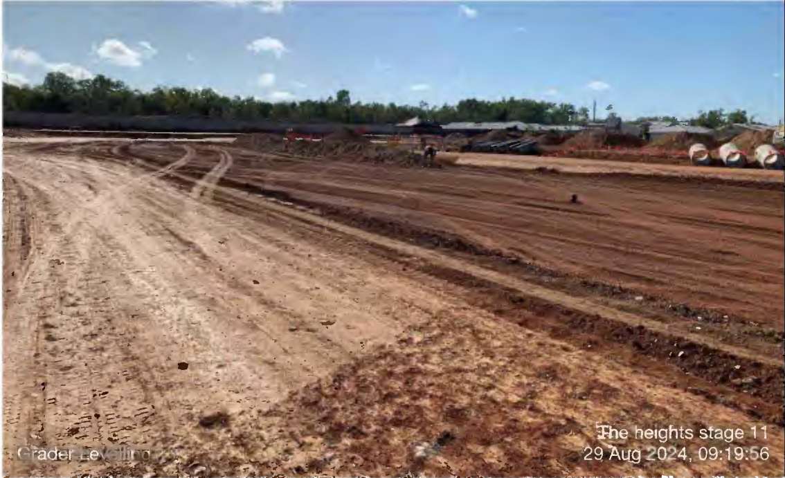
Photo 15 - The heights stage 11_2024-08-29_Grader Levelling_09-1 -
