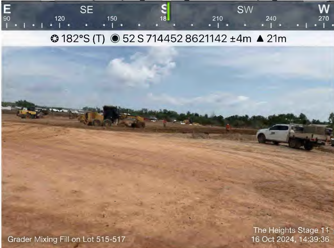
The Heights Stage 11_2024-10-16_Grader Mixing Fill on Lot 515-517
