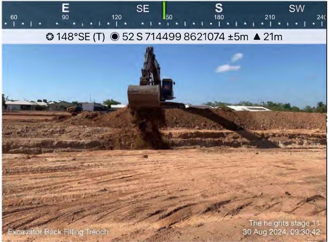
- The heights stage 11_2024-08-30_Excavator Back Filling Trench_
