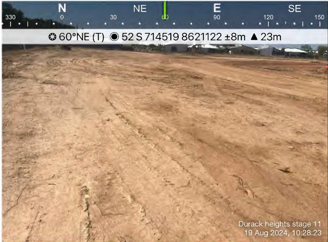
Photo 7 - Durack heights stage 17
