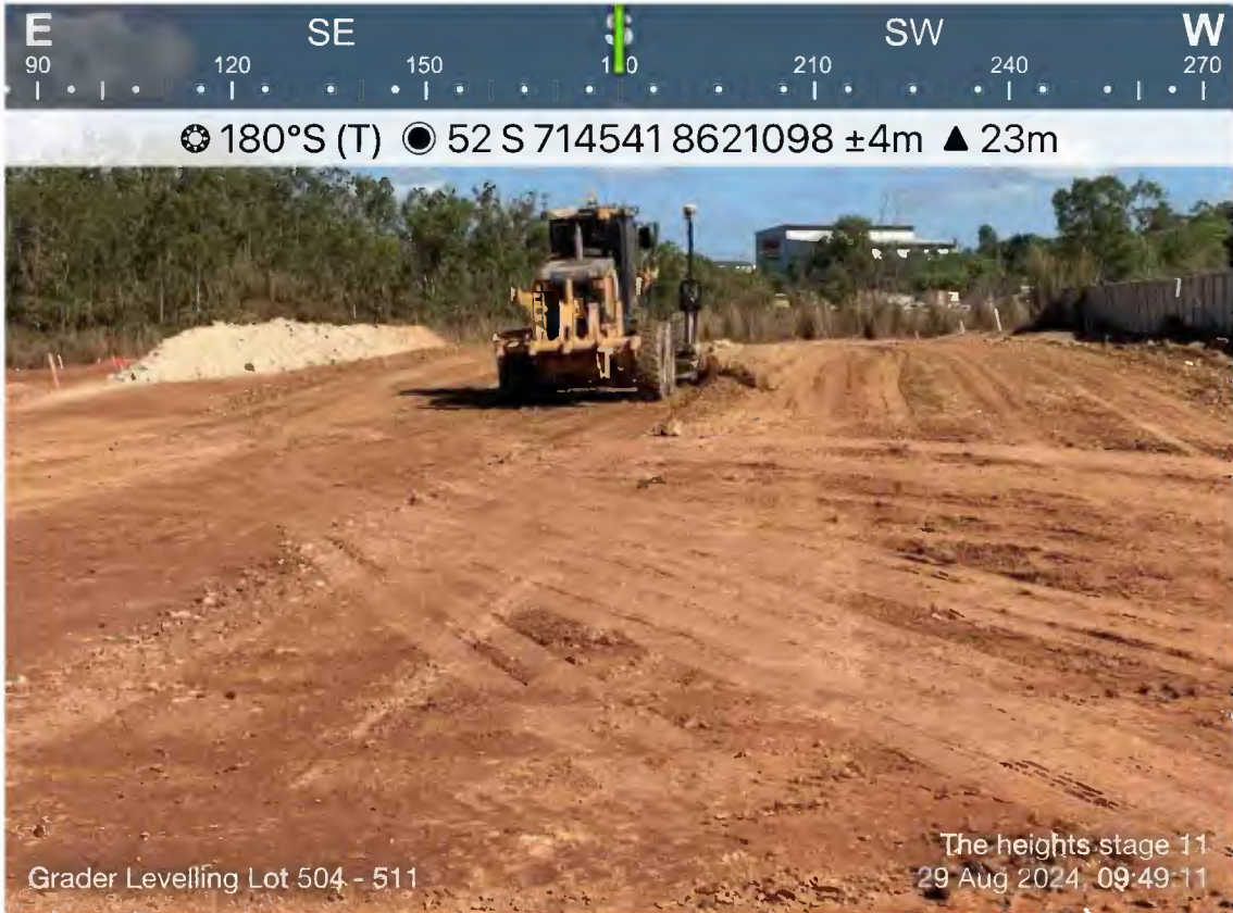
- The heights stage 11_2024-08-29_Grader Levelling Lot 504 - 511_
