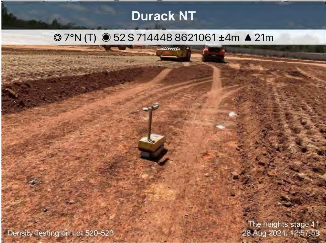
- The heights stage 11_2024-08-28_Density Testing on Lot 520-523_
