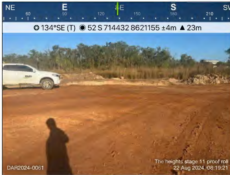
Figure 4: Site overview at Subgrade post-strip
