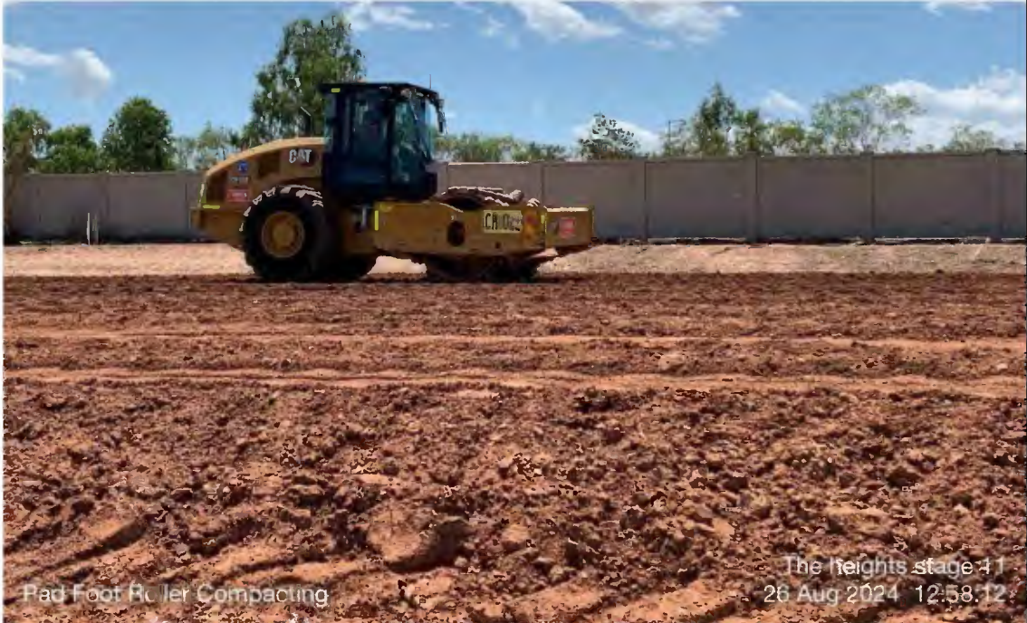
1 - The heights stage 11_2024-08-26_Pad Foot Roller Compacting_1
