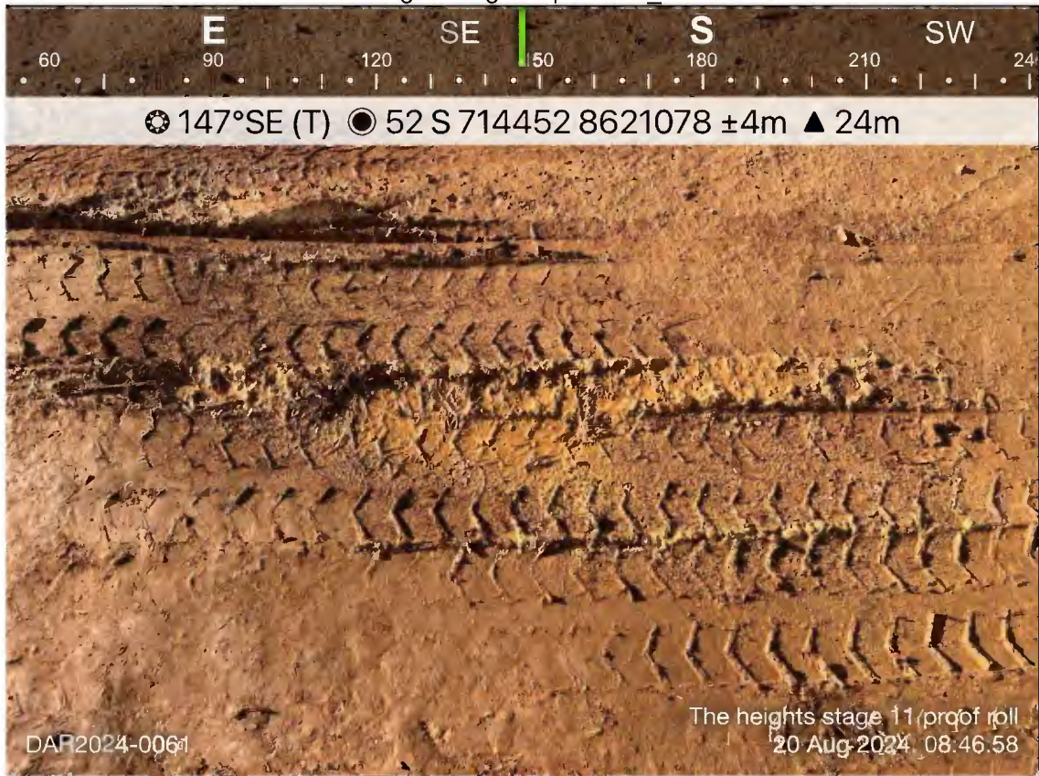
Photo 12 - The heights stage 11 proof roll_DAR2024-0061 2
