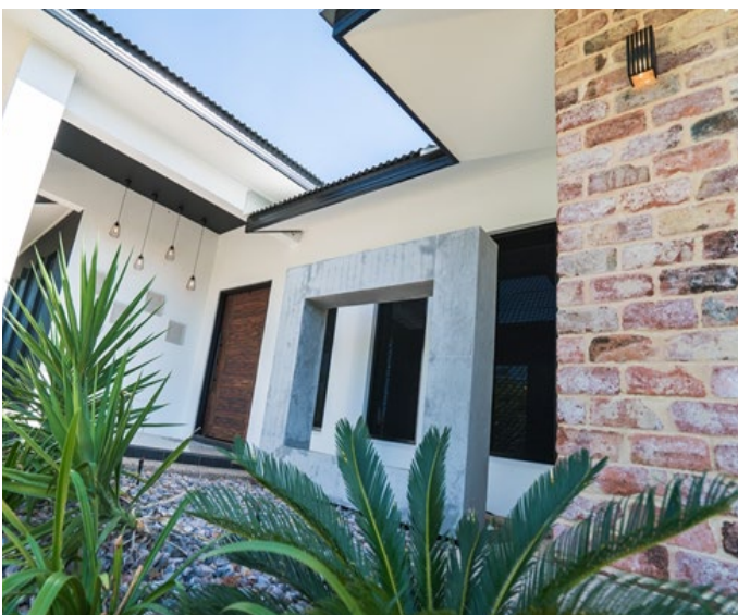
Above: The front façade must include at least two different wall materials
